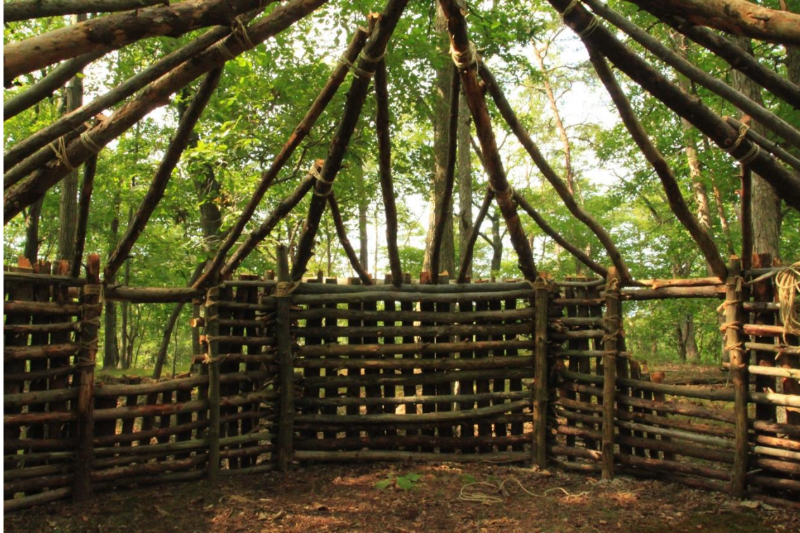
Figure 2: This is the completed foundation, using dead logs from the area.
